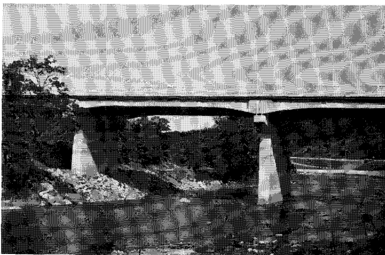
Fig. 5 Naugatuck River Bridge.
