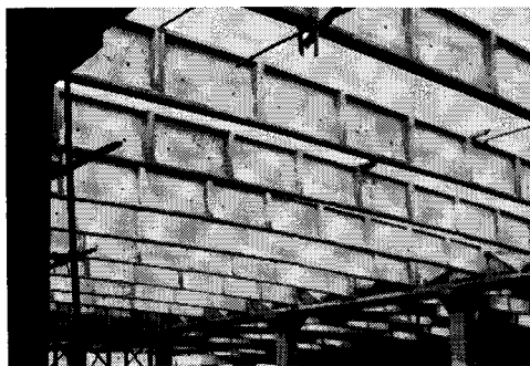
Fig. 12 Elemental beam for the French Kodak plant.
